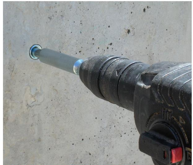
Anchor being set with SDS setting tool.
